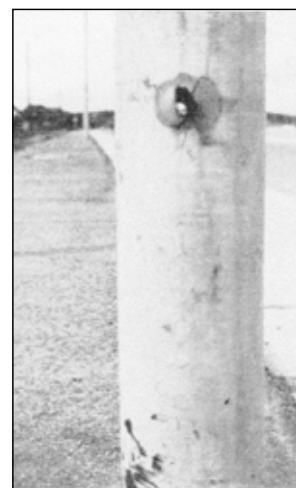
A 20 mm projectile from a Madsen cannon has penetrated this steel mast.
